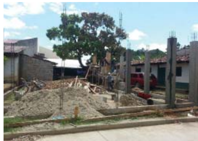
below: the posts for the walls
