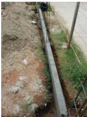
left: the foundation is laid
