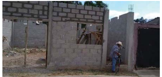
the walls are going up
