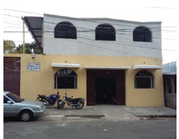
Unfinished 2nd floor; work has stopped until additional funds are raised to complete the addition.
